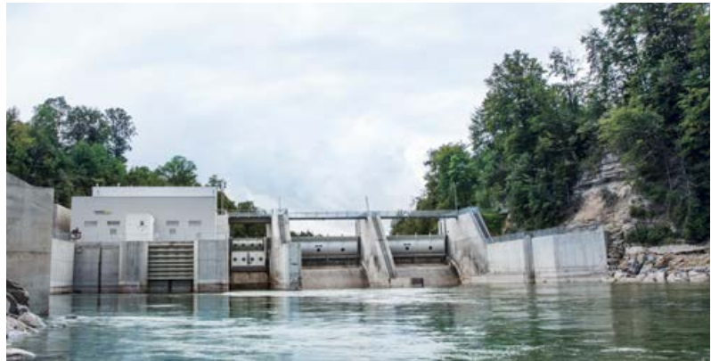
Hydropower plant Danzermühl in Laakirchen
