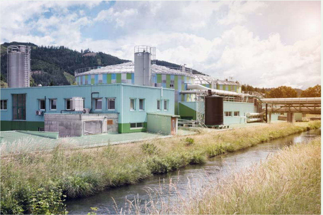
Water treatment at Zellstoff Pöls AG
