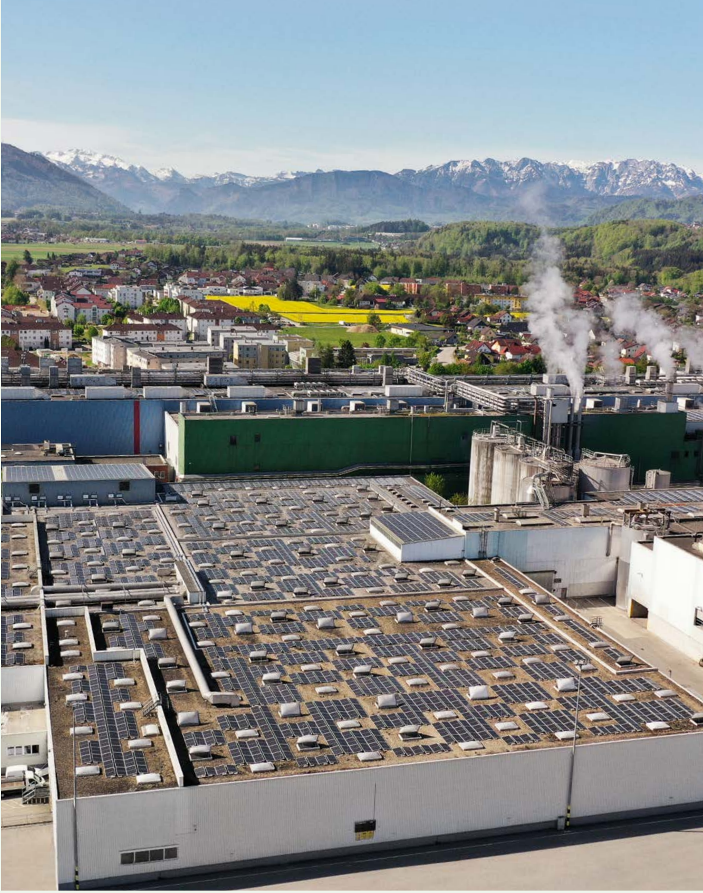
One of Austria's largest rooftop photovoltaic systems on the roofs of Laakirchen Papier AG.
