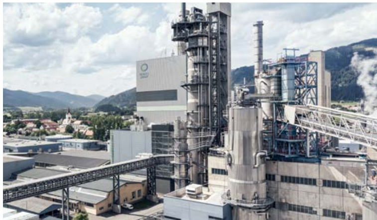
Ongoing optimization work in Pöls
