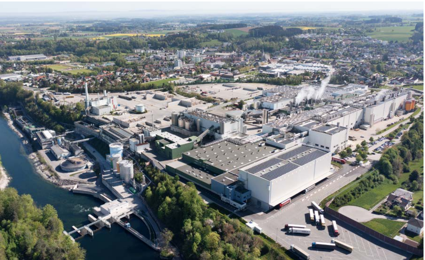
Focus on renewable energies: In Laakirchen, the hydropower plant and photovoltaic system together produce 47.6 GWh of electricity per year.
