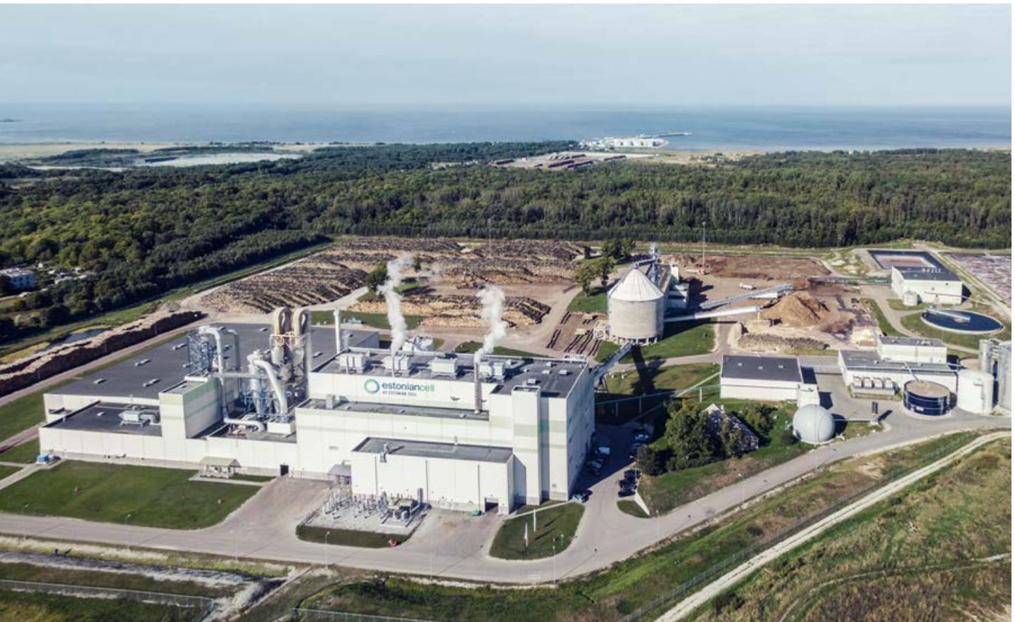
EUR 205 million was invested in the Estonian Cell construction work.
