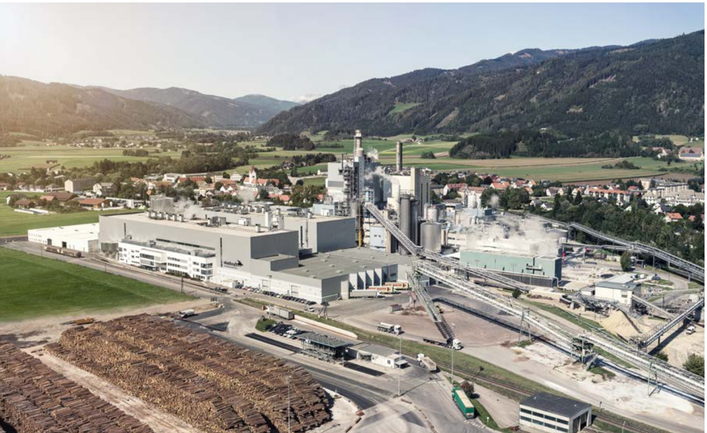
Around 460,000 metric tons of pulp are produced in Pöls every year.
